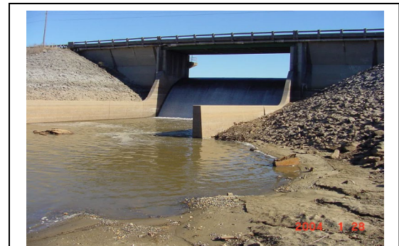
Figure 2-8. Acworth Sub-impoundment, Ungated Spillway
