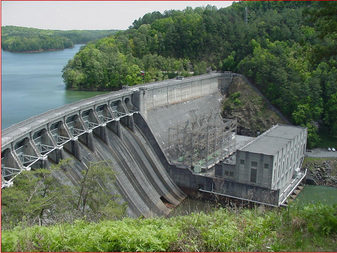
Allatoona Dam and Lake
