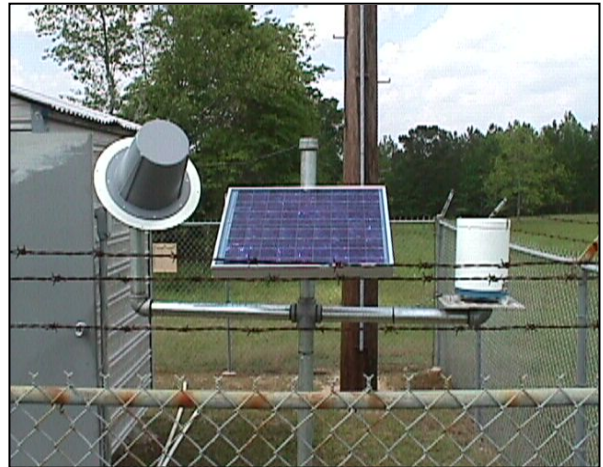
Figure 5-2. Typical field installation of a precipitation gage
