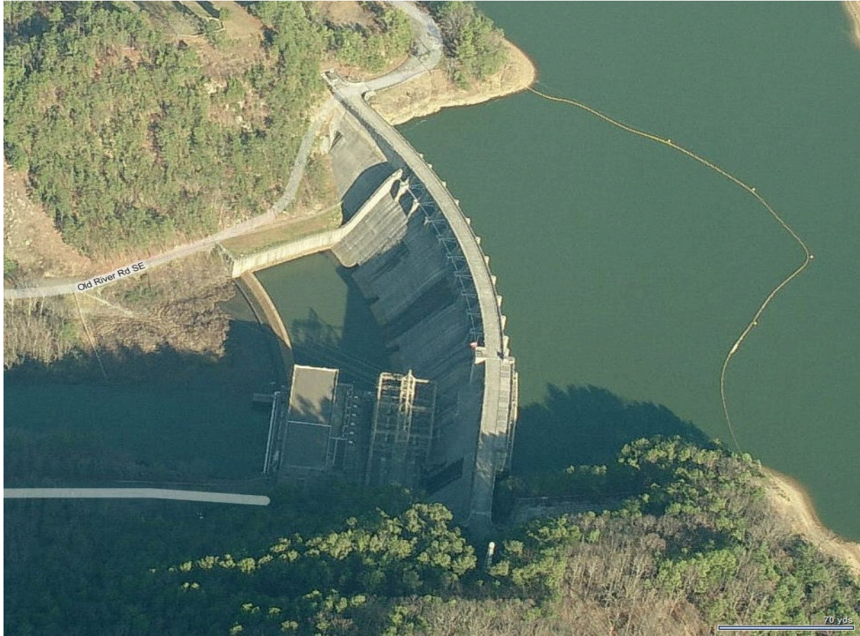
Figure 2-1. Allatoona Dam and Lake
